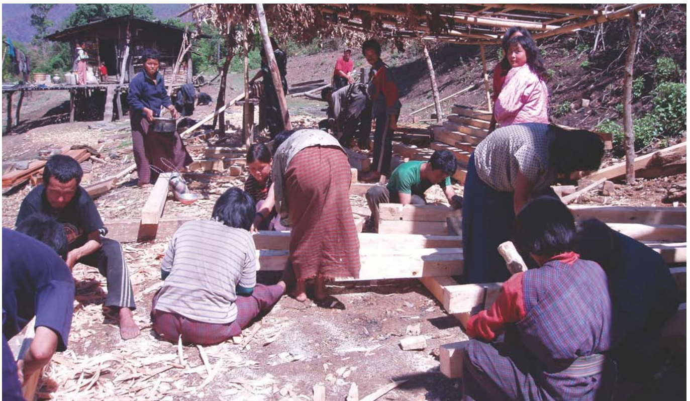
Community members of Rukha village, Athang Gewog jointly constructing a house, 2007.
